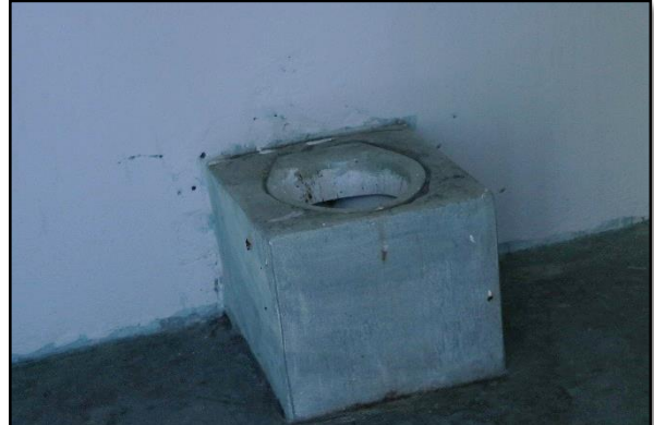
Figure 21 Toilet provided for use by detainees in the cells
