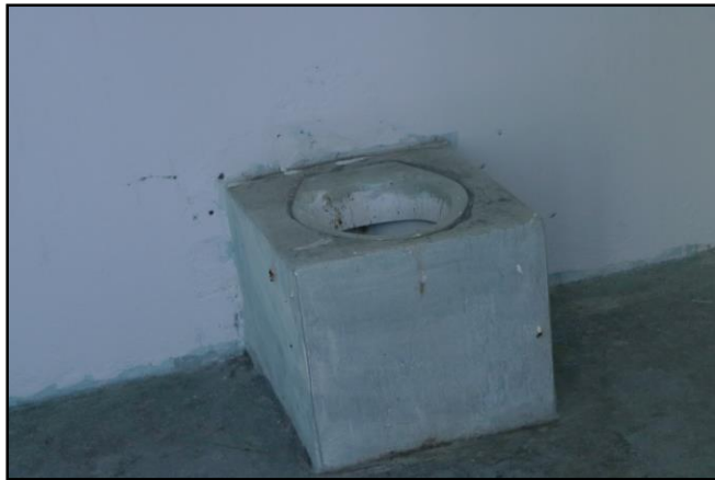
Figure 16 Toilet in holding cell at the Chaguanas Police Station
