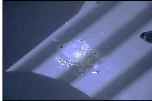
Figure 30 Place in suite where stainless steel stool was uprooted
