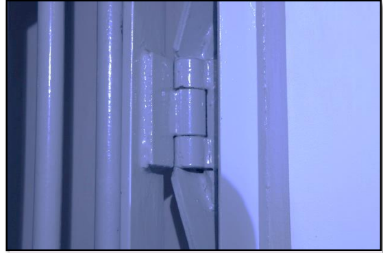
Figure 27 Redesigned hinges of the cell doors
