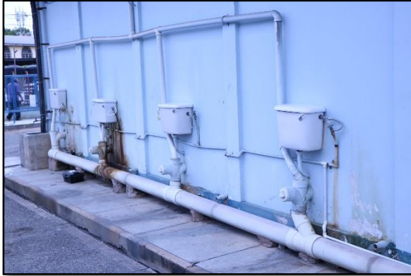
Figure 20 The tanks for the toilets in the cells located outside the Chaguanas Police Station
