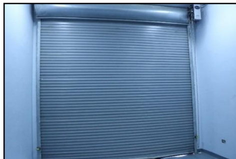
Figure 34 Gateway for access into the Vehicle Reception Area
