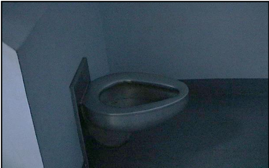
Figure 40 Toilet inside cell at the Besson Street Police Station
