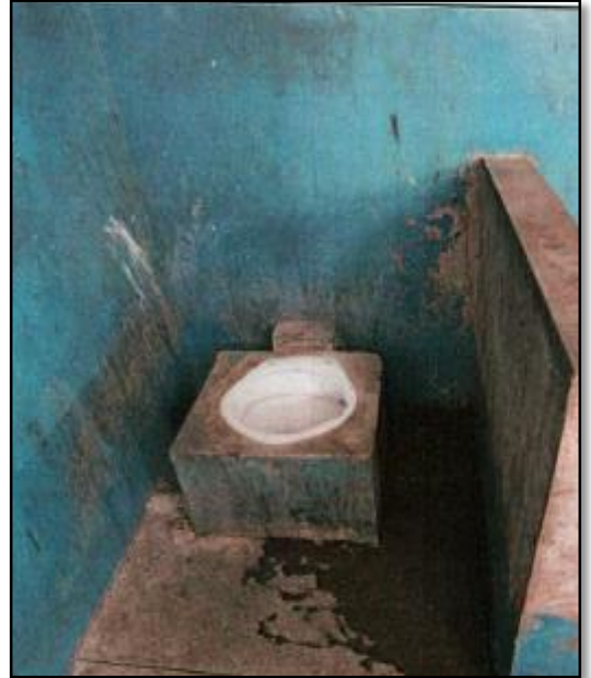
Figure 7 Toilet inside the holding cell at the Scarborough Police Station
