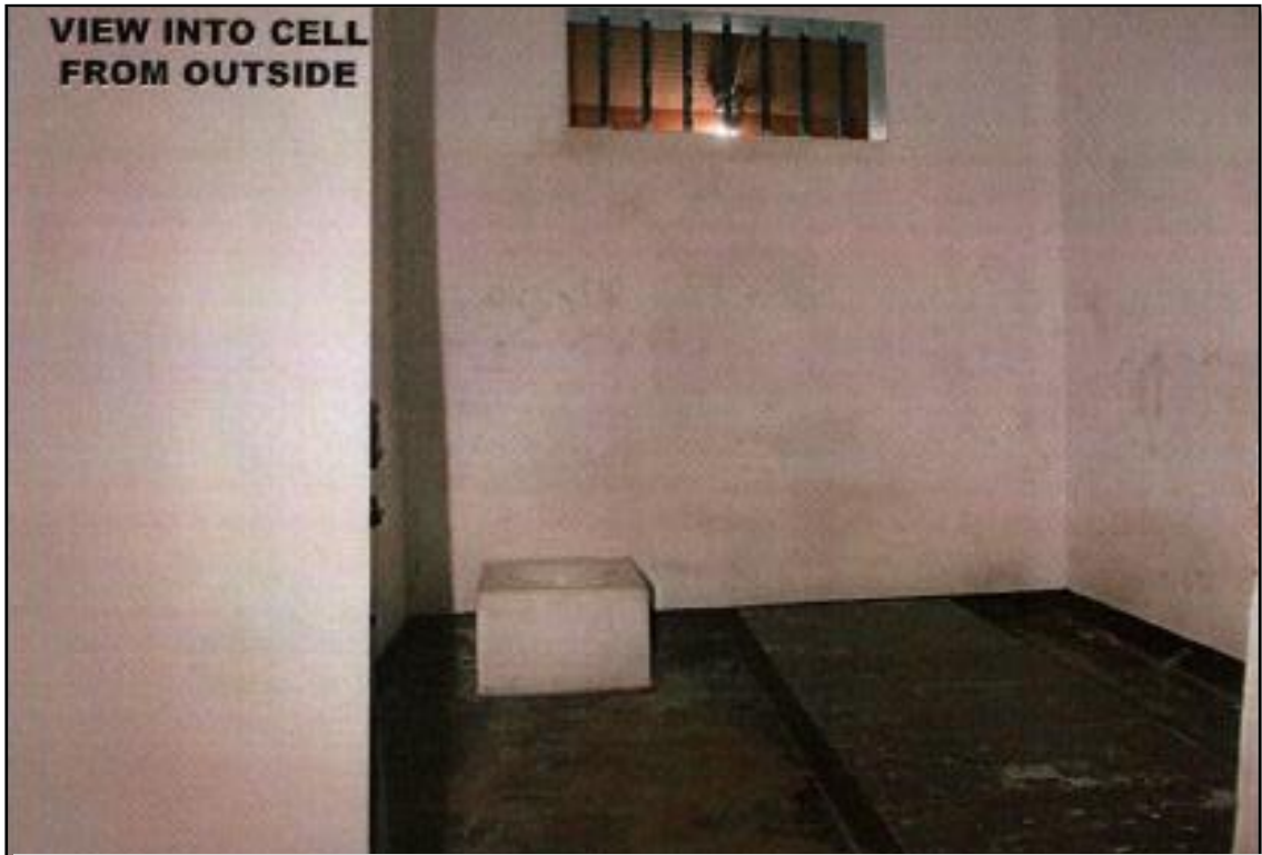
Figure 5 Holding cell at the Charlotteville Police Station, Tobago
